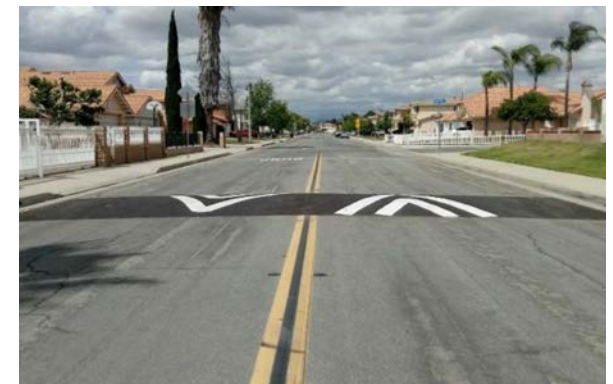
Speed humps are a common traffic calming measure in residential areas.
