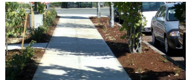
Low Impact Development practices like bioretention and porous paving help retain groundwater and capture storm water runoff.
