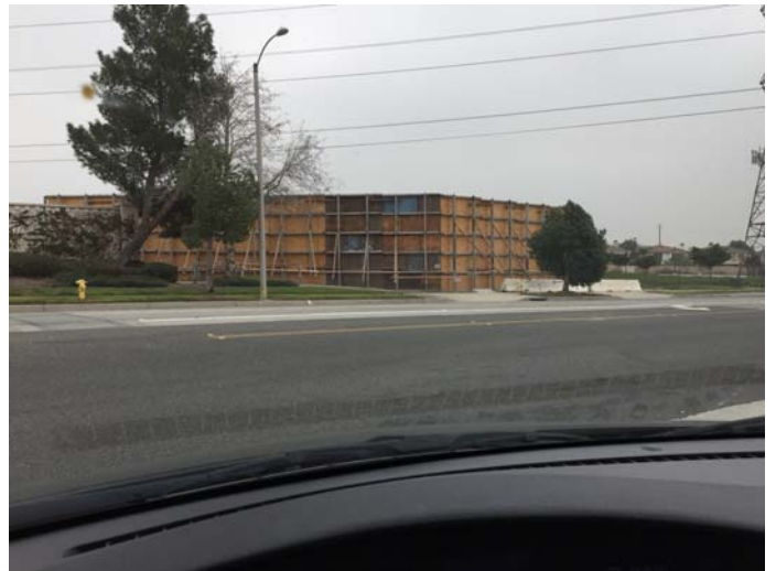
K-Rail Plywood & Acoustic Material
