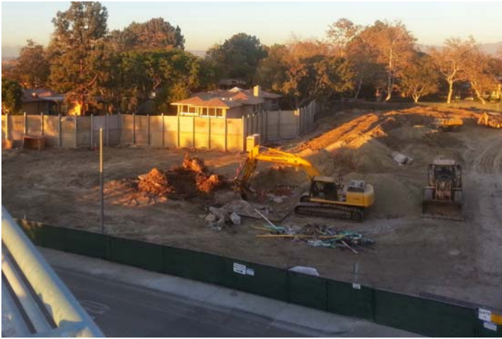
Pillar & Acoustic Material
