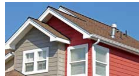
Rake and Eaves Overhang
